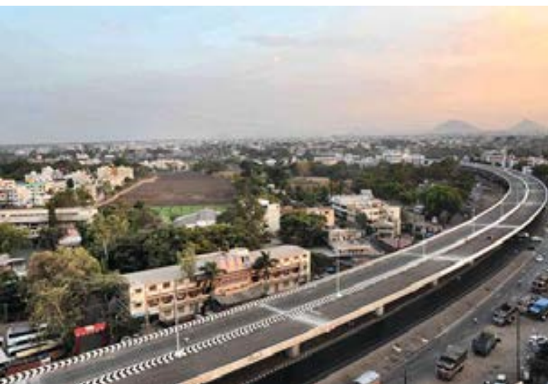
An Elevated Corridor sweeping over a city – one of L&T's many road development projects.
