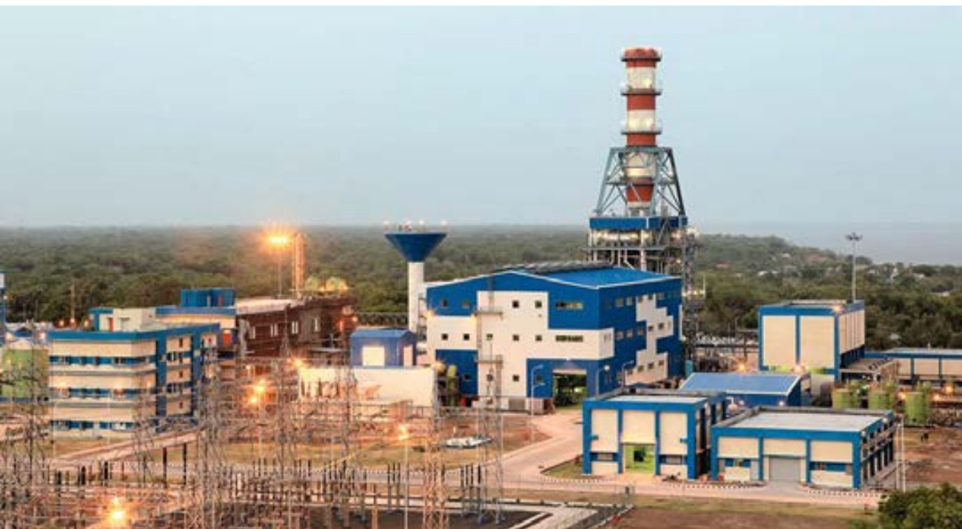
On EPC basis, L&T undertook the 375 MW single-shaft combined cycle power plant project for Gujarat State Electricity Corporation at Dhuvaran in Gujarat.
