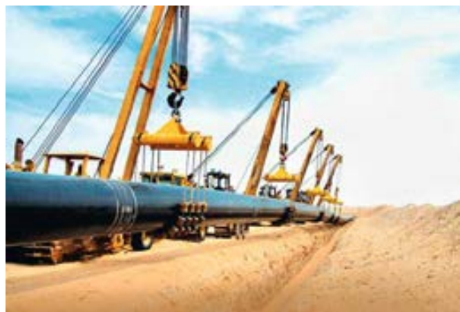
52"x 107 km Habshan-Ruwais-Shuweihat Gas Pipeline Project for GASCO, Abu Dhabi (UAE).
