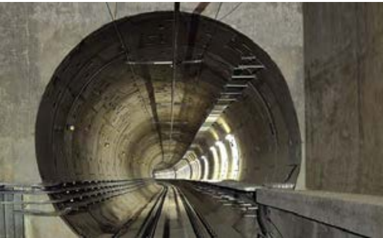
An underground section of the Chennai Metro.
