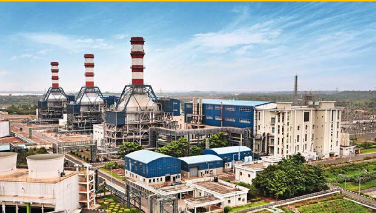
Natural-gas-fired combined cycle power plant built by L&T at Vemagiri in Andhra Pradesh.
