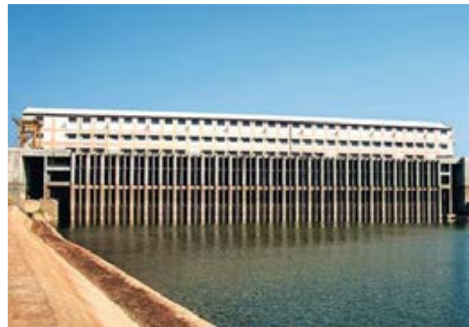
Hanamapur lift irrigation project, Karnataka.
