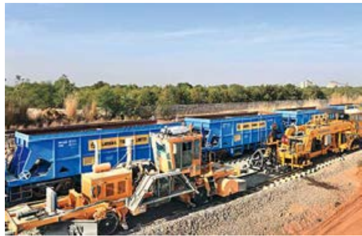
L&T has deployed a new track construction machine capable of laying 2 km of tracks per day - setting a benchmark in high-speed rail construction.
