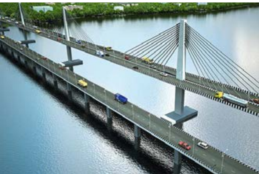
Across River Mandovi in Goa, L&T is building one of India's longest cable-stayed bridges.
