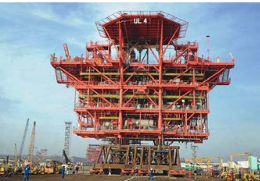
Load-out of offshore modules for ADMA-OPCO, Abu Dhabi from Sohar Yard in Oman
