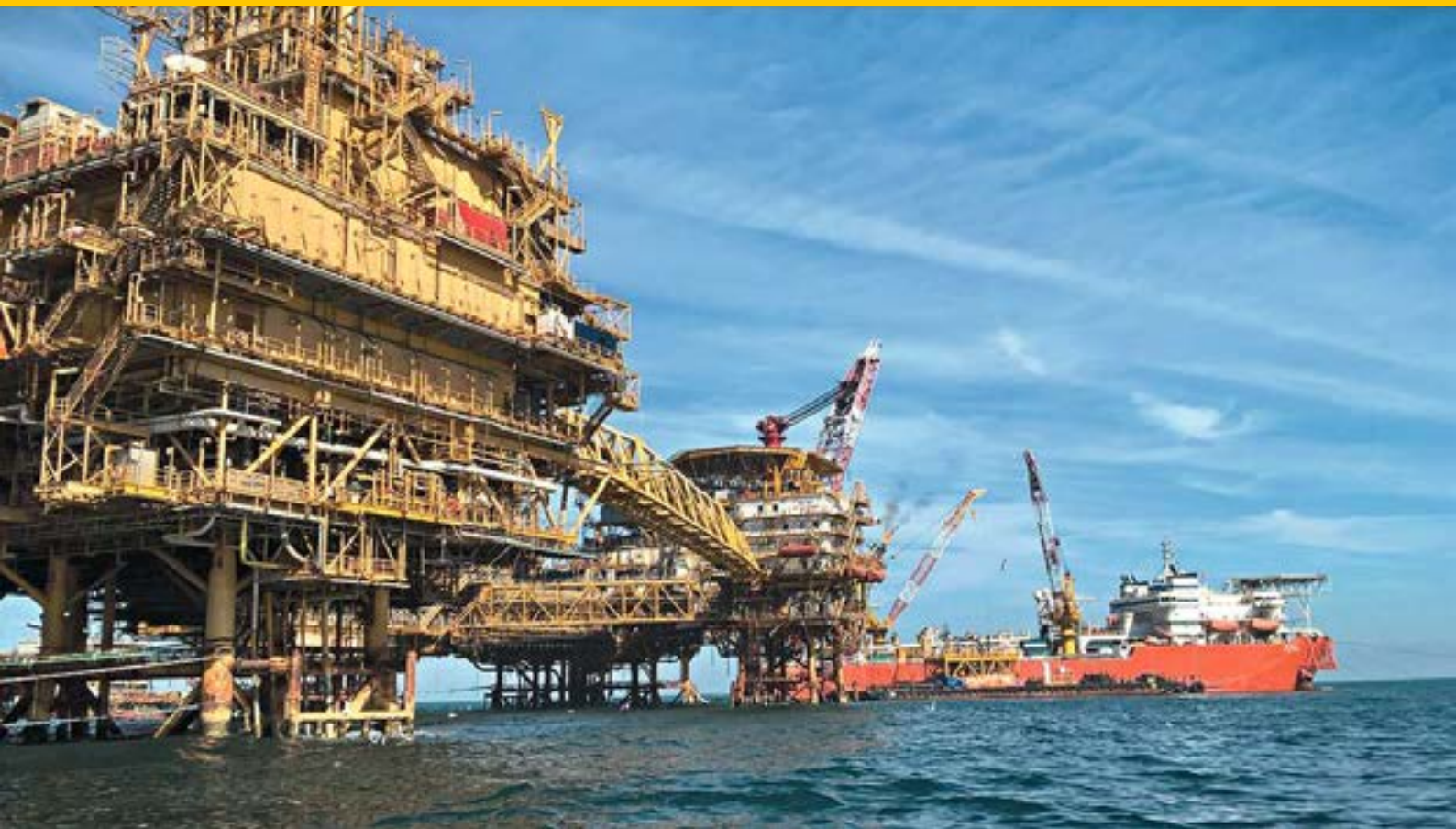
One of many mega-offshore projects executed by L&T's hydrocarbon business. Picture shows captive heavy-lift-cum-pipelay vessel LTS 3000 in the background.
