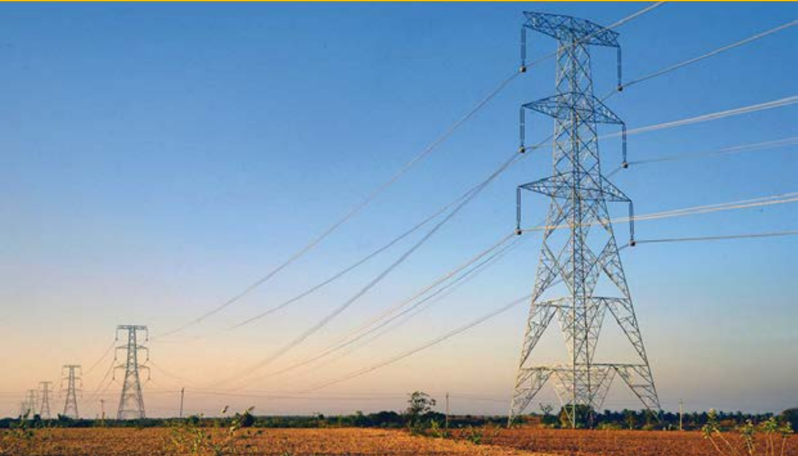
Kudgi Power Transmission Line project, Karnataka.
