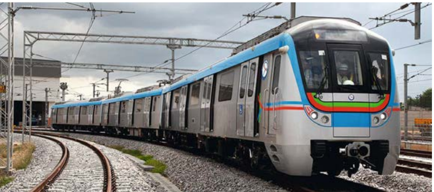
The Hyderabad Metro project is the world's largest public-private-partnership in the urban transportation sector.
