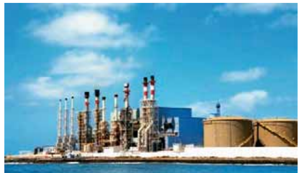
Desalination is helping the world supplement a vital resource. L&T's capabilities in the water sector include setting up of thermal desalination plants.
