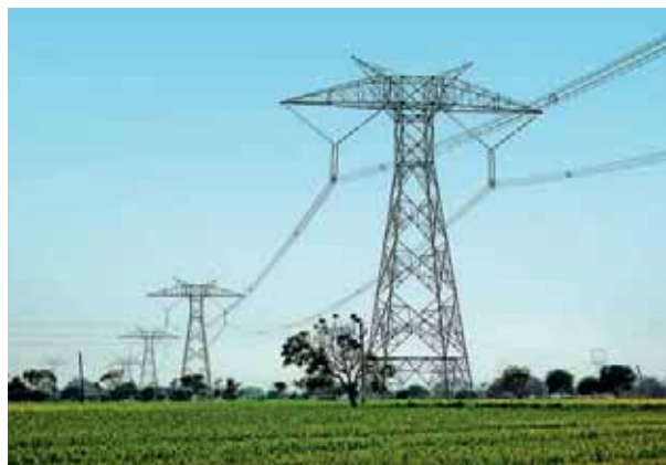
800 kV transmission lines between Nidhura and Agra.
