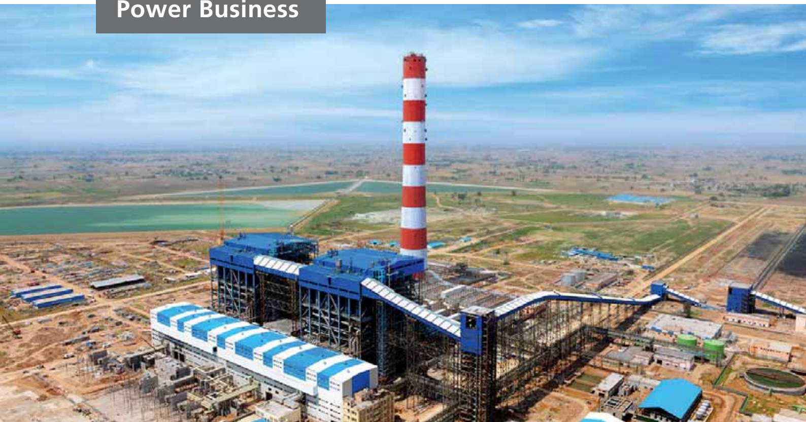
2x700 MW supercritical thermal power plant built by L&T on EPC basis for Nabha Power at Rajpura in Punjab. L&T's joint venture with Mitsubishi Hitachi Power Systems enables the power sector to access the advantages of world-class technology.
