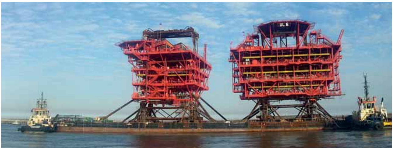
Topsides sail away from L&T Modular Fabrication Yard in Sohar, Oman for Nasr & Umm Lulu Development project of ADMA-OPCO, Abu Dhabi.
