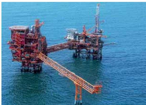
DDW1 Wellhead Platform & Process-cum-living quarters platform for GSPC installed off India's east coast.
