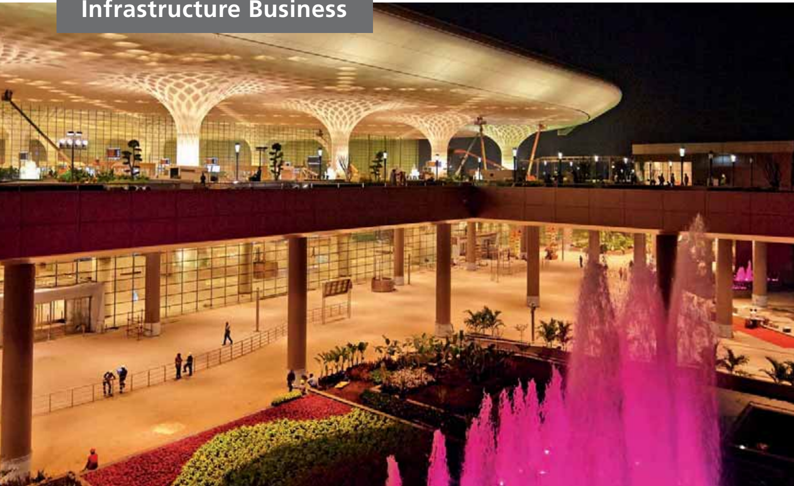
The new Gateway of India - Terminal 2 at Mumbai Airport. L&T has constructed several modern airports that include New Delhi, Bengaluru and Hyderabad in India. The Salalah International Airport in Oman is at an advanced stage of construction.
