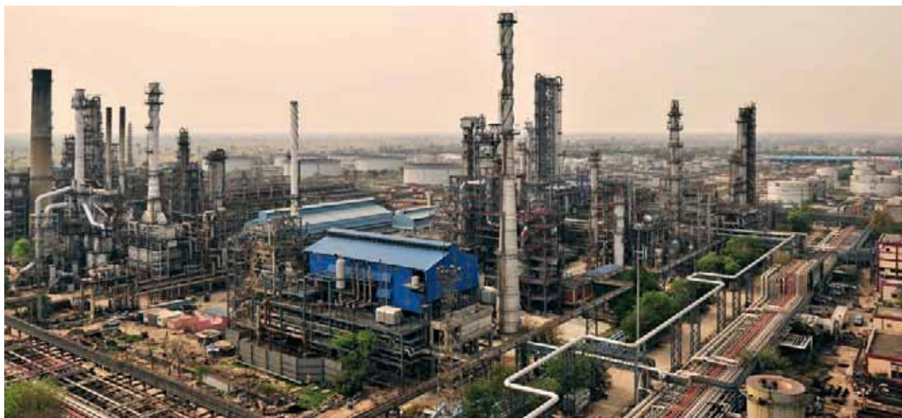
Motor Spirit Upgradation Project and Diesel HDS project with offsites & utilities executed for IOCL-Mathura refinery complex.
