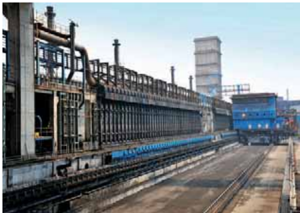
Coke oven battery executed by L&T for one of India's major steel plants.
