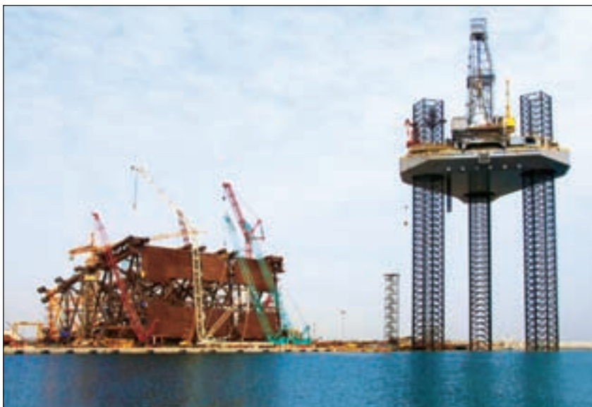
Jack-up drilling rig (right) for Lynemouth Drilling, U.K. and 13,500-tonne jacket for ONGC at L&T's Modular Fabrication Yard in Sohar, Oman.
