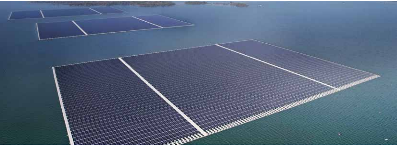
90 MW Floating Solar Project, Omkareshwar, Madhya Pradesh
