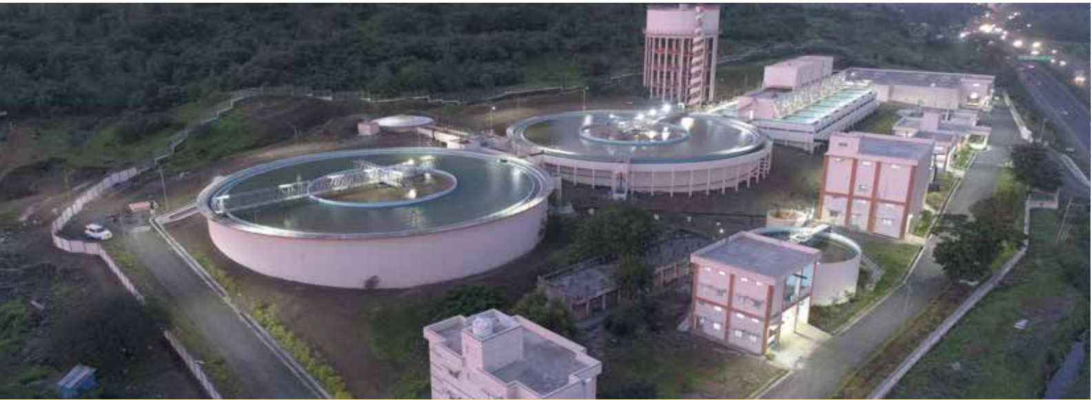
Water Treatment Plant at Nashik, Maharashtra
