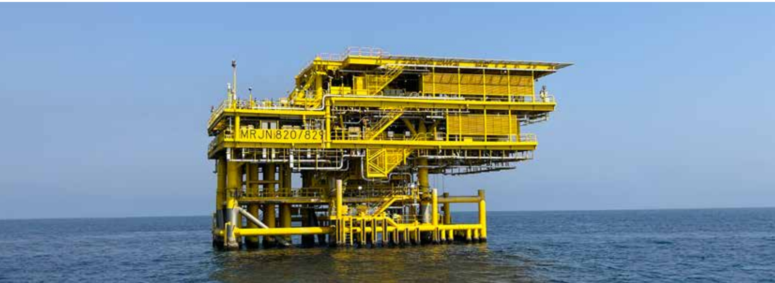
Oil Production Deck Module for Saudi waters
