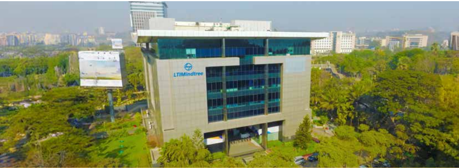
LTIMindtree Headquarters, Powai, Mumbai, Maharashtra
