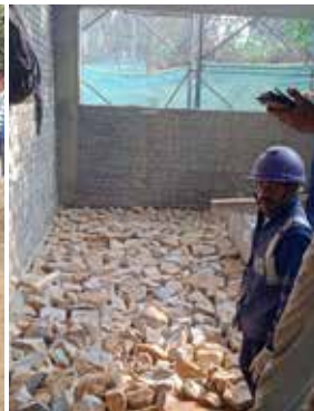
Reuse of Concrete Waste - structure pedestal, building floor, canteen benches
